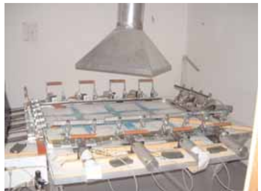
Local ventilation installed over stretching table at Technograph
